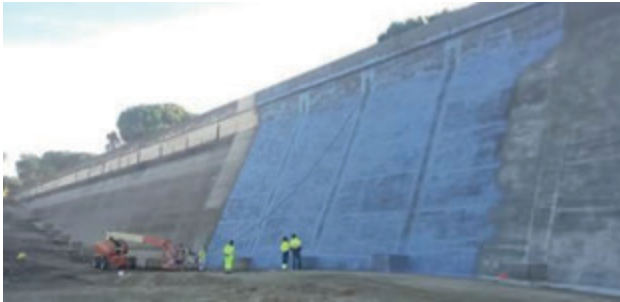
Repairing and waterproofing the San Juan reservoir (Madrid)
